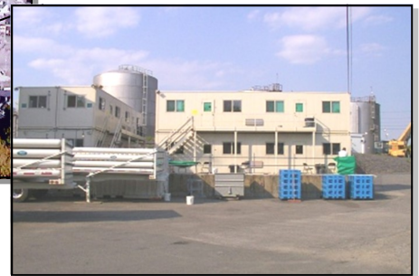
24' x 54' x 12' - 10,650 square foot Double wide construction with clear span capacity allows for open floor plan configuration.
